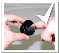
Lubricate internal bore.
