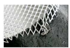
Attach the mesh to the grill surround with the supplied wire. This mesh may require some minor trimming to fit. Bend the edges of the mesh over the side and fasten it tightly with the supplied wire. The wire needs to be cut into several pieces, one for each mount point.
